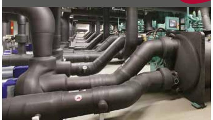
A flexible insulation with superior weathering characteristics and suitable for higher temperature applications of up to 150°C.
