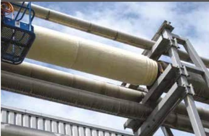
Pyrogel® XT-E is a high-temperature insulation blanket formed with silica aerogel applied to a reinforced non-woven, high-temperature matrix. Pyrogel® XTF has been specially formulated to provide exceptional protection against fire.
