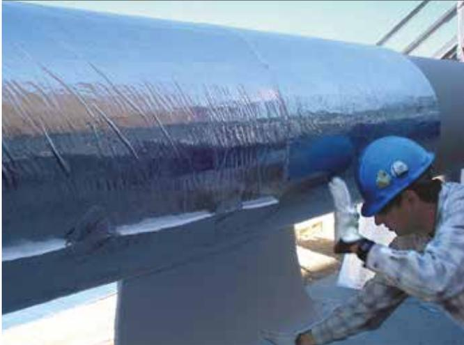
Cryogel® Z is a highly efficient low temperature Aerogel product with an integral vapour barrier facing.
